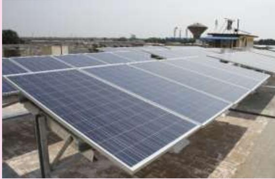
**100 KWp** ON-Grid Solar Rooftop PV System is provided at roof top of ICF Shell Administrative Building & IT Centre. Annual Potential Generation would be 1.2 Lakh units which will eventually reduce CO2 emission by 96 ton/year
