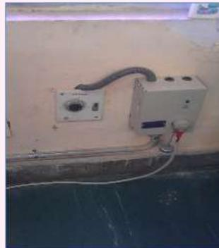
Occupancy Sensor have been provided in Officer's Chamber to switch off automatically Air Conditioners and Room Lights when the Room is unoccupied
