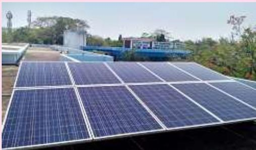
**15 KWp** On-Grid solar PV system installed at ICF Hospital roof top
