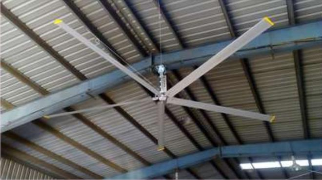
One no of High Volume Low Speed (VFD) 24ft sweep ceiling fan of capacity 1.5kw 5 blade has been installed in dispatch shed of furnishing division. The fan rotates at 65 RPM.
