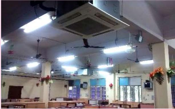
The conventional Window/Split Air conditioners are replaced with the state of the art Variable Refrigerant Flow (VRF) Centralized Air Conditioning System in both Shell and Furnishing Offices, which consume 40% less Energy
