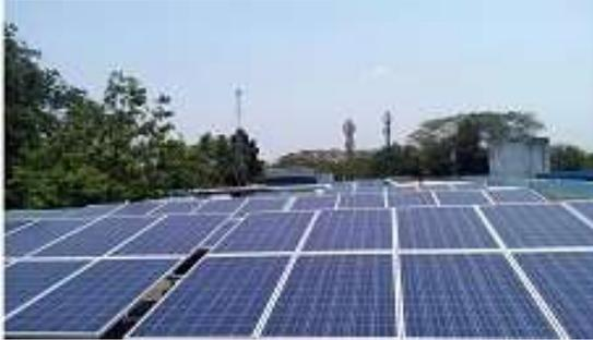
**10 KWp** On-Grid Solar roof PV system is provided at ICF Higher Secondary School, On an annual average it almost covers entire electricity requirement of the school
