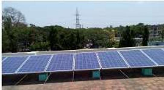
**3 KWp** Off-Grid solar PV system installed for illuminating approach road of LHB shed
