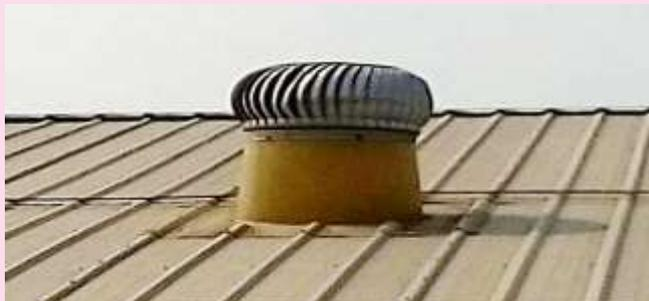
Turbine Air Ventilators which operate on natural draft without Electrical Power have been installed in Workshop Roof Tops to exhaust hot gas emanating from Welding Operation, Furnace etc.
