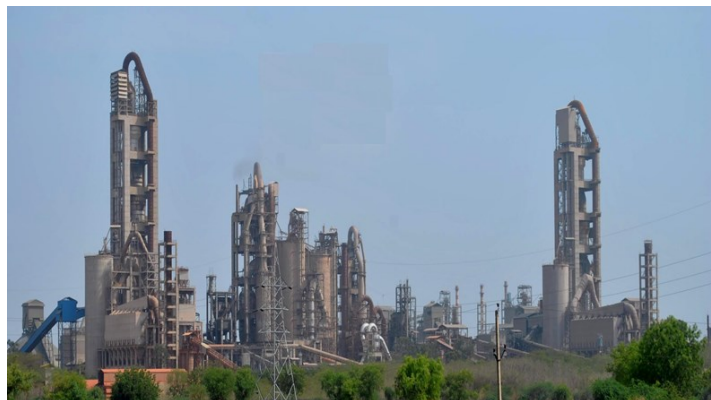
Vasavadatta Cement Plant, Sedam Unit
