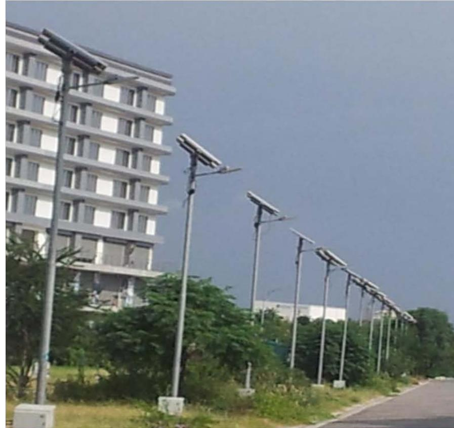
Street light are battery operated, Battery got Charged during day times & used in night
