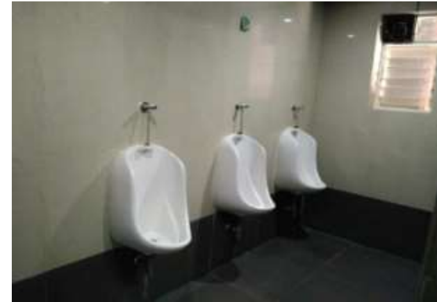
Push type taps provided for urines
