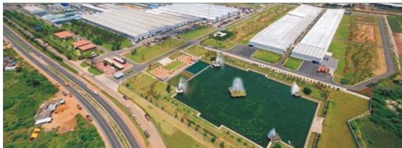
Water reservoir for storing rain water
